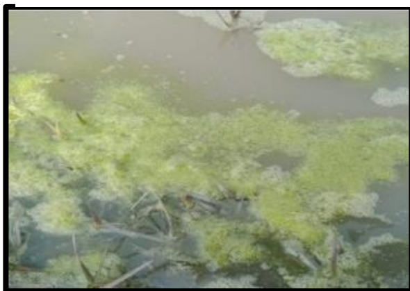
Figure 10. Algal infestation in a roadside drainage waterway
